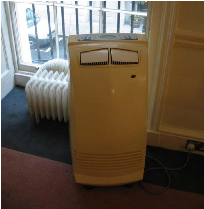
Photo 7: Stand alone air-conditioning unit
